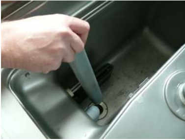
Remove the overflow pipe
