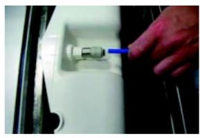
.....and remove water sump from evaporator basin
