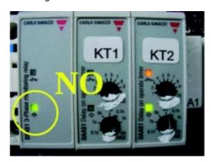
6. Correct wiring is shown by both LEDs Green and Orange steady ON together.
