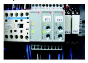
**NOTE**. In case on any temporally Ice maker trip OFF (not alarm) due to NO/LOW water pressure, bin full, ice spout switch activation unit stops by only keeping drive motor operating for 18' in order to clear evaporator by ice. KT2 delay relay LEDs steady ON (orange and green) during this delay.
