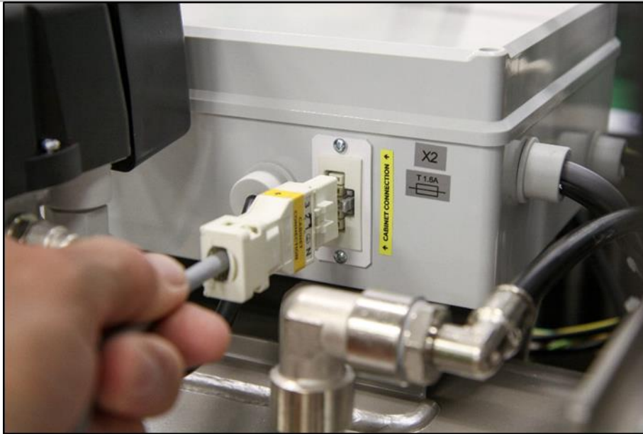
Fig. 18: Connect the cabinet to the compressor
