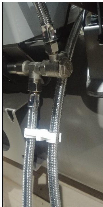
Fig. 12: Location of the first double clip
